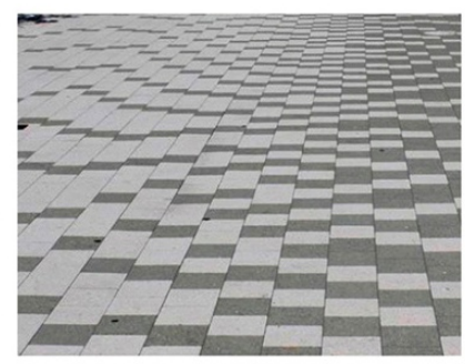
HIGH TIDE PATH PAVING
